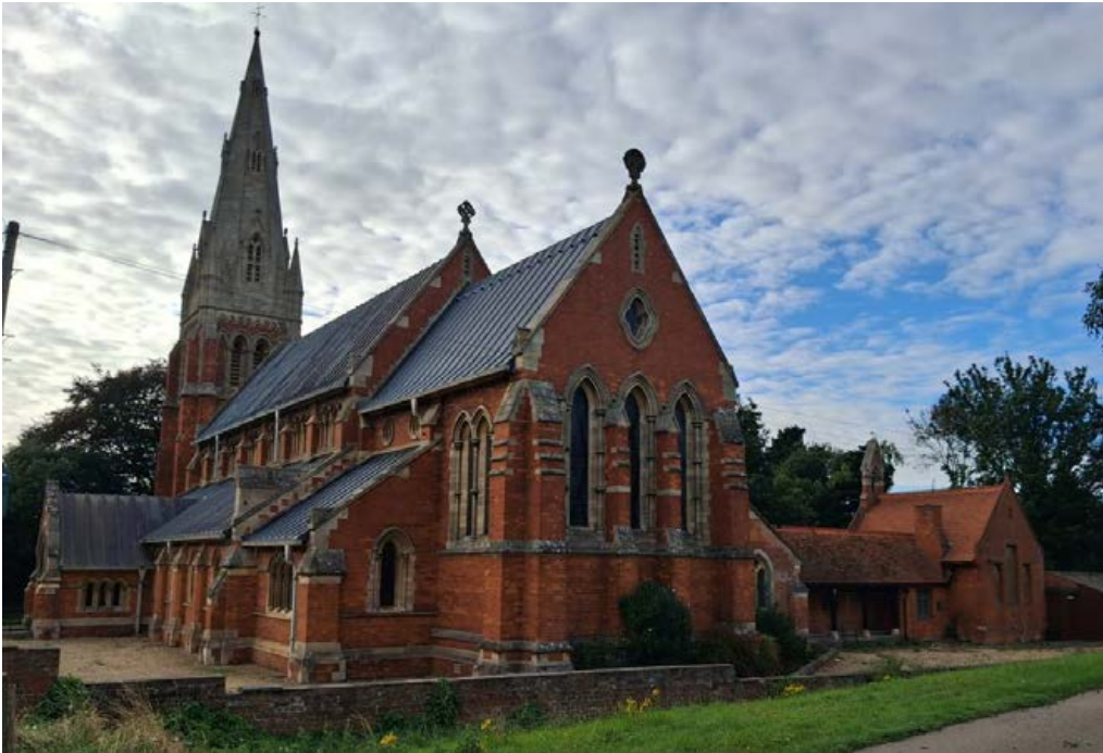
Plate 50: Grade I Listed Church of St Paul including attached schoolroom (1306702), Spalding. Grade II* Listed Vicarage is behind the church
