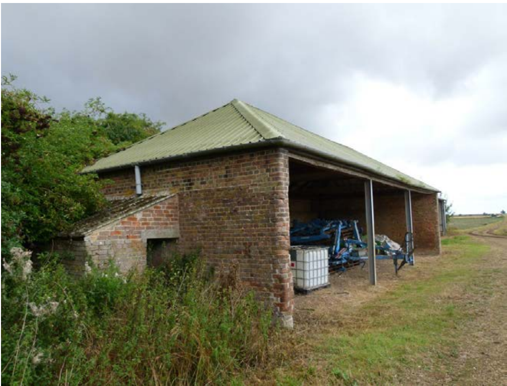
Plate 23: Cart shed at Lodge Farm (MLI123864), Solar Development Area, field A-1
