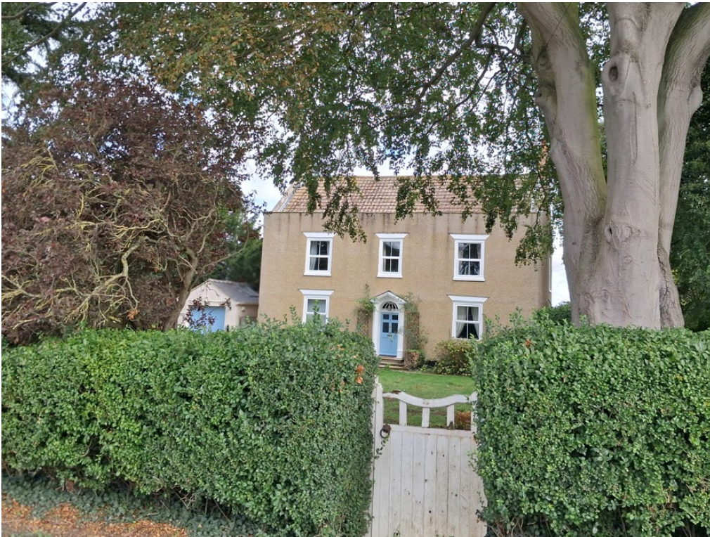
Plate 61: Listed Beech House (1147482), Broadgate
